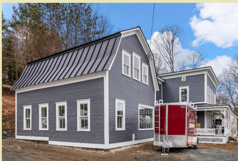
61 N. Bradford Street – After (Source: Village Ventures)
