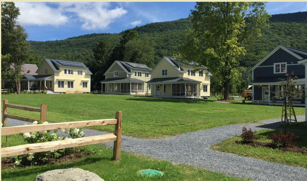
Photo: Cottage Court in Bristol Village, VT Cohousing (Vermont Integrated Architecture)
