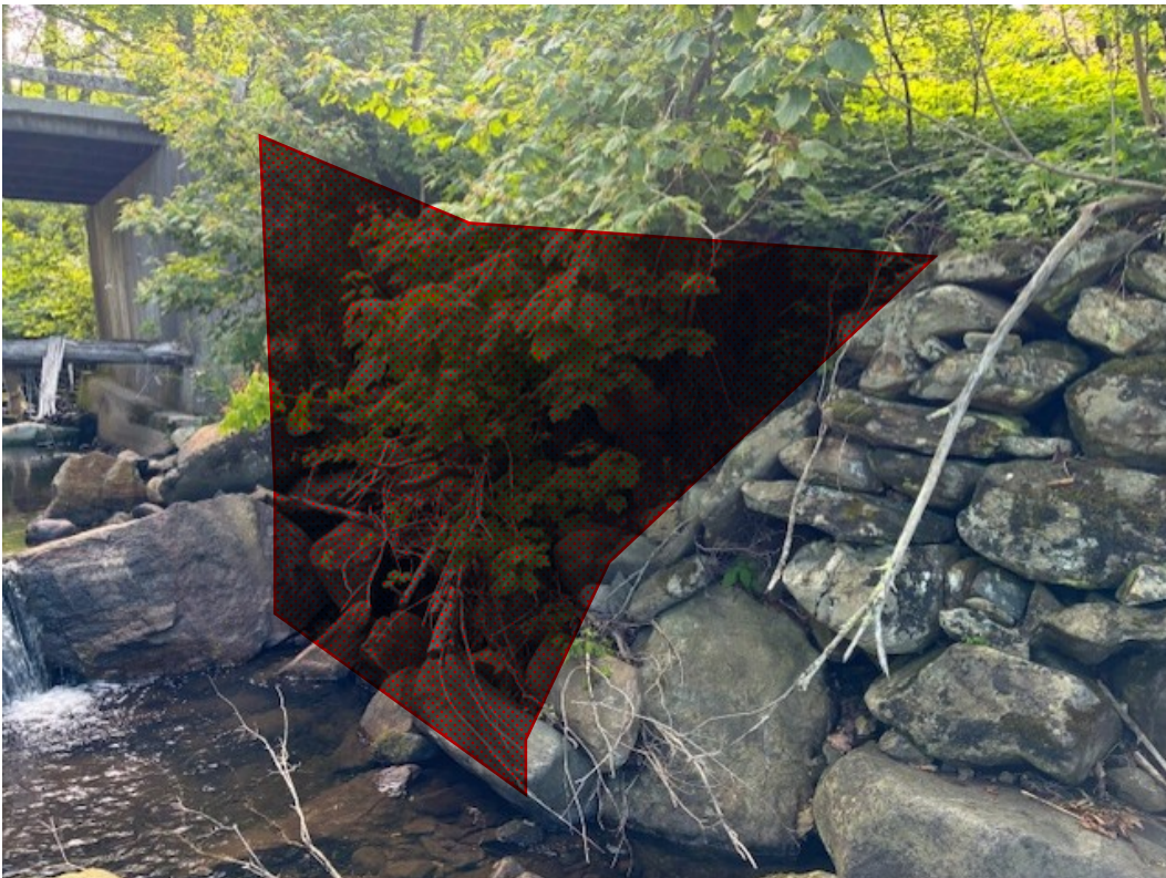
Photo 4: Looking at damaged wingwall from opposite bank. Tie into existing wall on right side of photo. Taper wall up to match top of existing concrete abutment.
