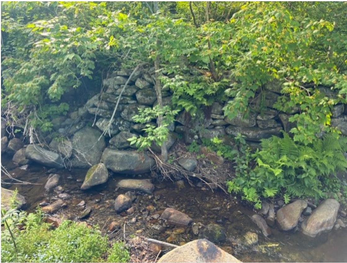
Photo 5: Existing wall to match into. Intent is to match existing wall as much as possible in color. Sizing of new rock should 3-4' at base and as wall is built up in height size can reduce to 18"-3'. Looking for tightly stacked wall.
