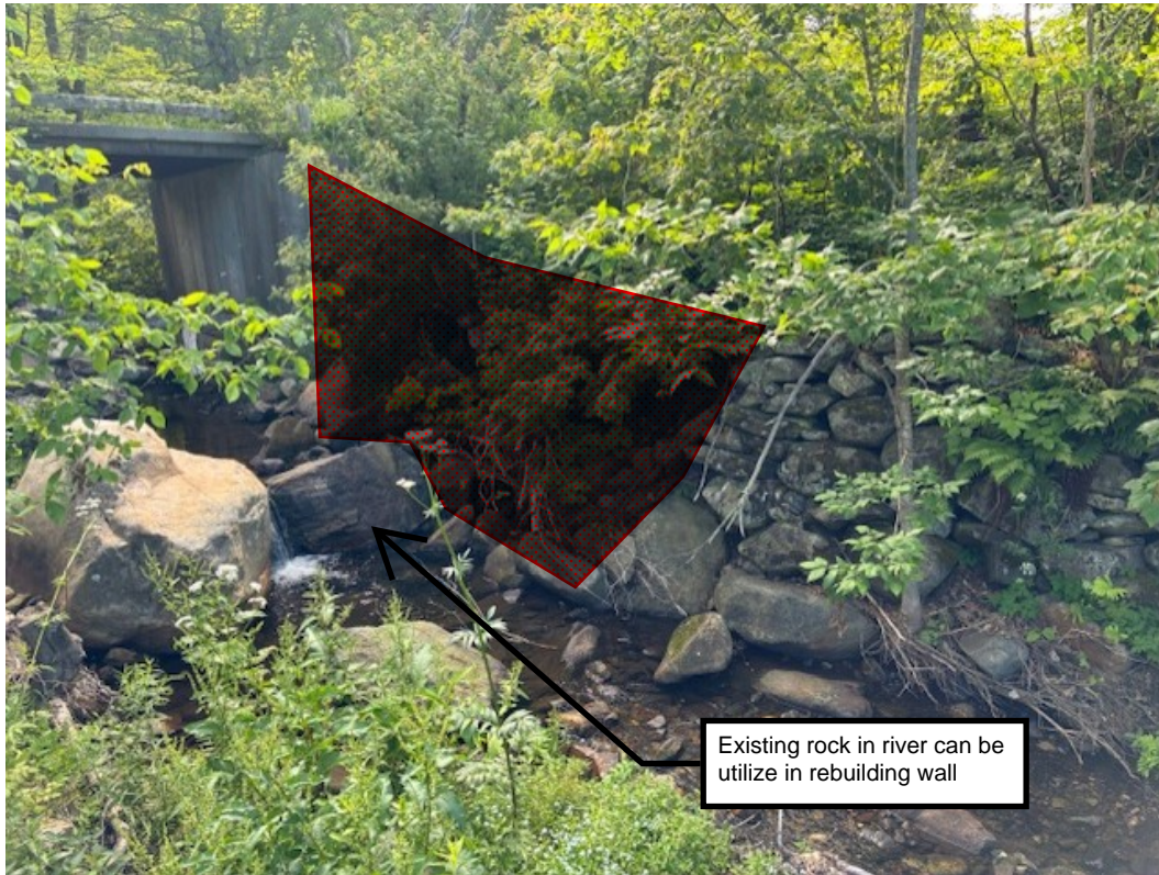
Photo 3: Looking at damaged wingwall from opposite bank
