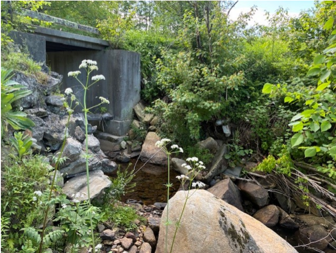
Photo 1: Looking at damaged wingwall from opposite bank
