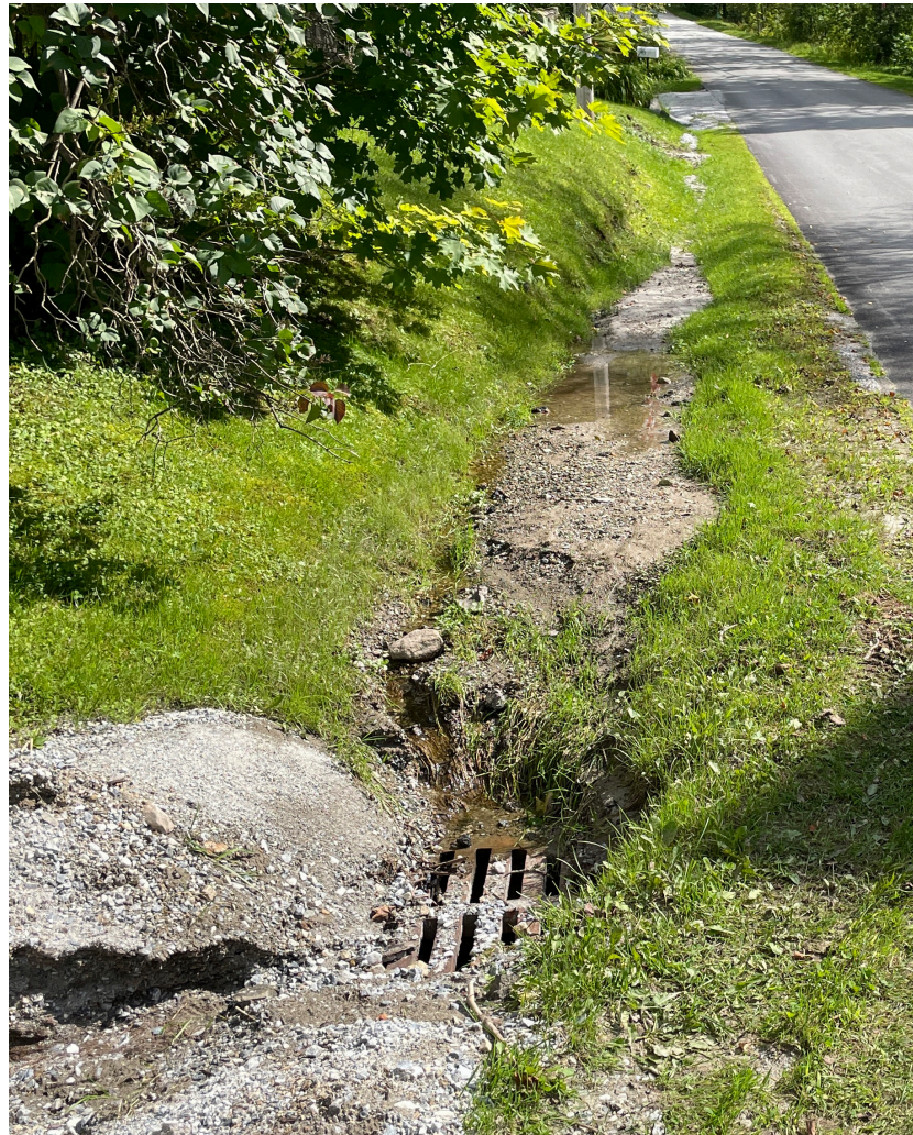
Stormwater Issues. The driveway of the church on Church Street is commonly washed out from an outlet pipe located uphill (above) and the resulting washout is carried down to the intersection where gravel deposits collect and create a hazardous condition for vehicles attempting to stop on the hill (below); Catch basins in the village are commonly clogged with gravel and debris, hampering proper drainage (right).
