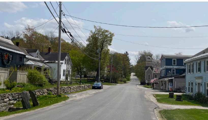
Belmont Road Obstacles. Existing utility poles and open stormwater inlets (see detail below) are creating obstacles within the town right-of-way, making it difficult to plow in the winter or use this area for parking.
