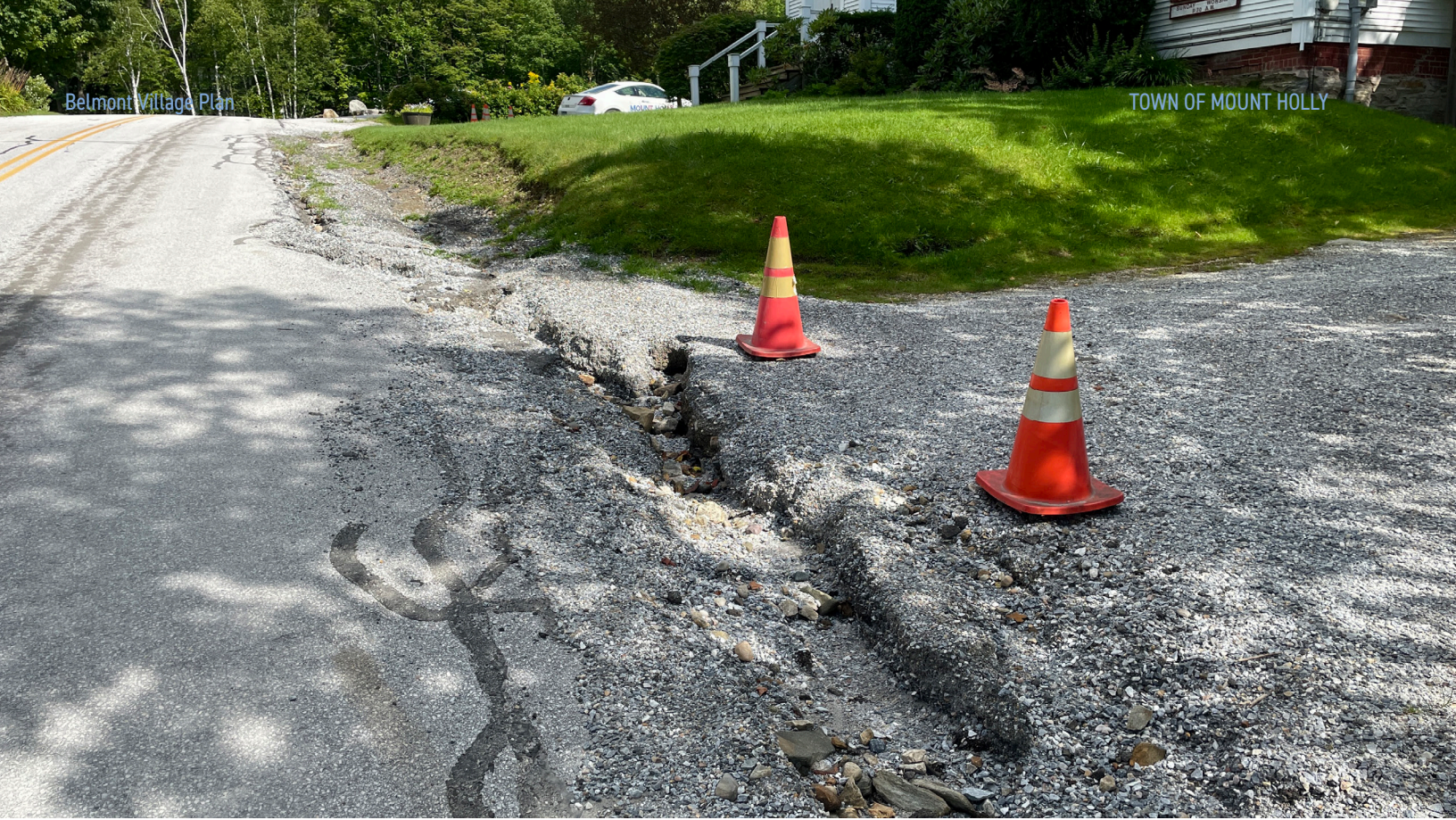
Stormwater Issues. The driveway of the church on Church Street is commonly washed out from an outlet pipe located uphill (above) and the resulting washout is carried down to the intersection where gravel deposits collect and create a hazardous condition for vehicles attempting to stop on the hill (below); Catch basins in the village are commonly clogged with gravel and debris, hampering proper drainage (right).
