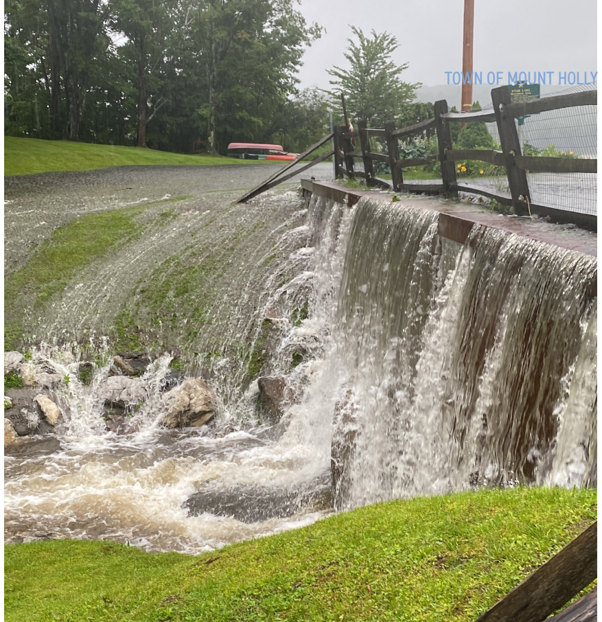
July 9, 2023 Storm Flooding. Overflow from Star Lake pouring through the spillway (above); Star Lake outflow at Belmont Street surcharging beyond its design capacity (left); Overflow and flooding at Belmont Road where the stone and concrete culvert passes underneath the road. (below).
