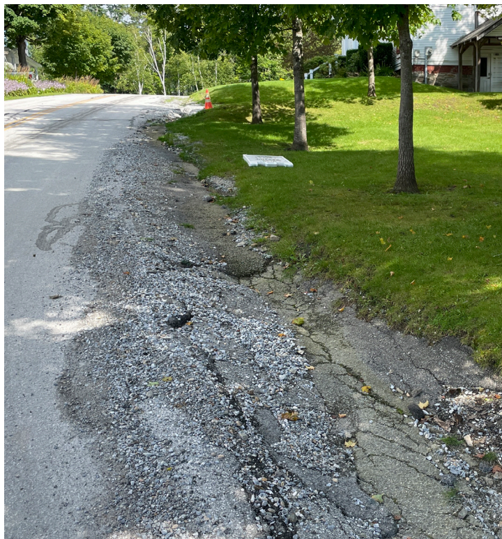
Stormwater Issues. The driveway of the church on Church Street is commonly washed out from an outlet pipe located uphill (above) and the resulting washout is carried down to the intersection where gravel deposits collect and create a hazardous condition for vehicles attempting to stop on the hill (below); Catch basins in the village are commonly clogged with gravel and debris, hampering proper drainage (right).
