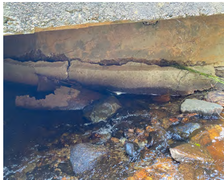
July 9, 2023 Storm Damage. Damage and repairs underway at Belmont Road, where the surcharging culvert compromised the road integrity (above); Photo inside the existing culvert where structural damage and failure is clearly visible (below).
