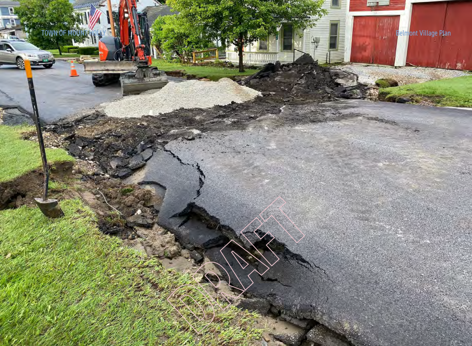
July 9, 2023 Storm Damage. Damage and repairs underway at Belmont Road, where the surcharging culvert compromised the road integrity (above); Photo inside the existing culvert where structural damage and failure is clearly visible (below).
