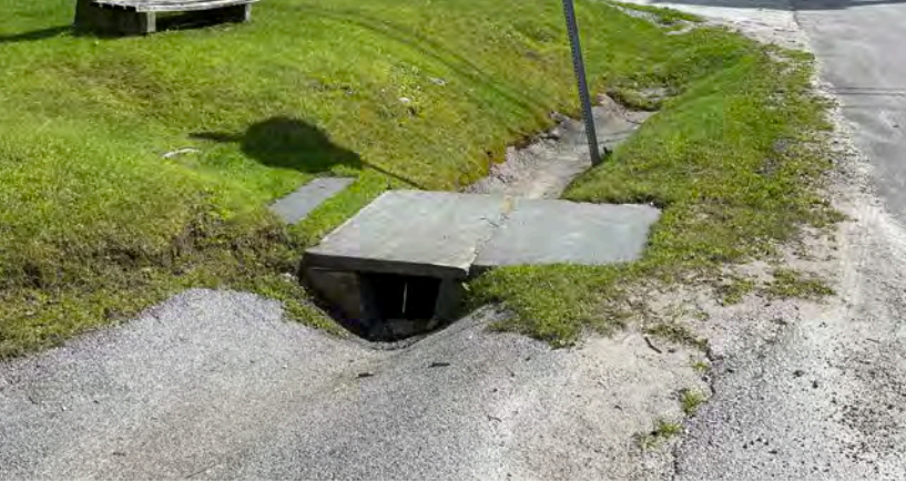
Stormwater Inlet. Open stormwater inlet interferes with on-street parking potential and can be a hazard for pedestrians.
