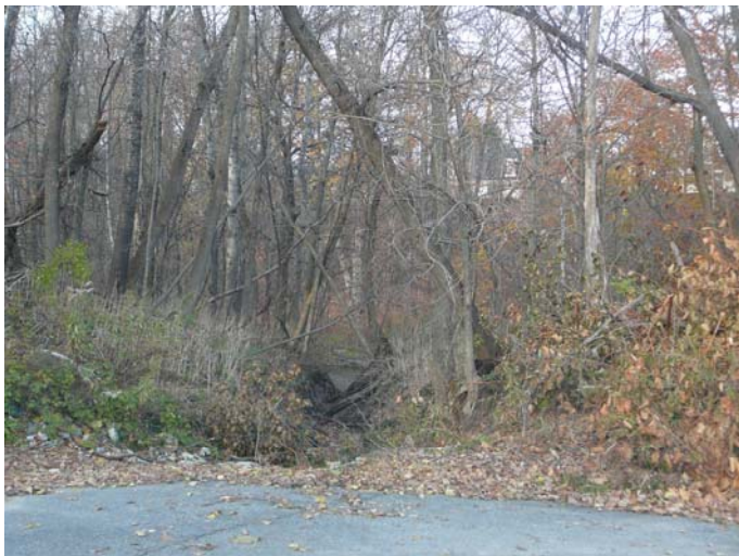
Figure 17. RB stormwater channel from commercial plaza near downstream end of reach M34 has developed into an erosional gully that has deposited gravels and sands in the Black River channel. View to the northeast from corner of parking lot toward the river. Trees along the side slopes of this gully are leaning in toward the channel due to bank collapse. 8 November 2007.
