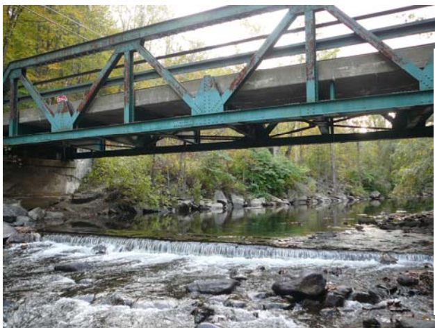
Figure 18. Remnants of historic dam below Mill Street bridge crossing, 1 October 2007. This dam remnant was indexed as a grade control, but is not expected to have significant impoundment effects or disrupt sediment continuity to a significant degree.
