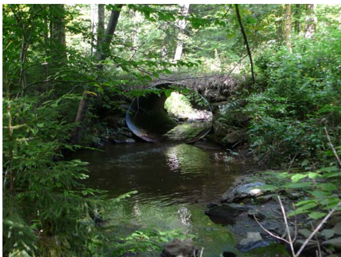
Figure 29. View upstream, to bankfull constricting culvert crossing under Reading Pond Road, Segment B, M41T6.02S1.02, Reading Pond Brook, 4 September 2009.
