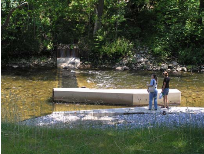
Figure 14a. Inflatable bladder/weir and flume for measurement of Black River flows associated with Okemo Mountain snow making project. Located on the Black River (reach M34) in Ludlow. Dam not inflated at time of observation, 29 May 2006. View to northeast from RB.
