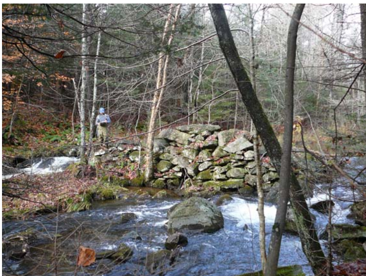
Figure 10. Remnants of breached dam at bifurcation in Patch Brook channel. View upstream, M40T5.03 Segment B, Patch Brook; 29 October 2009
