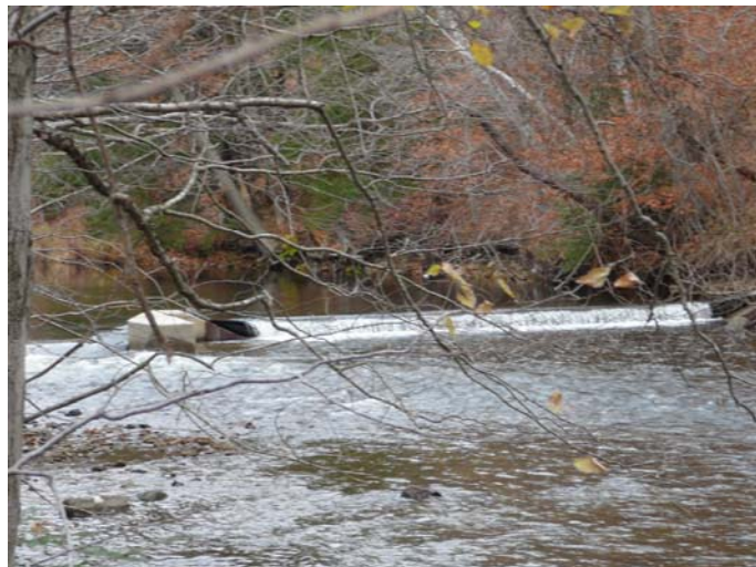
Figure 14b. Inflatable bladder/weir and flume; bladder (dam) inflated at time of observation, some spillage over the dam/weir evident. View upstream from RB. 8 November 2007.
