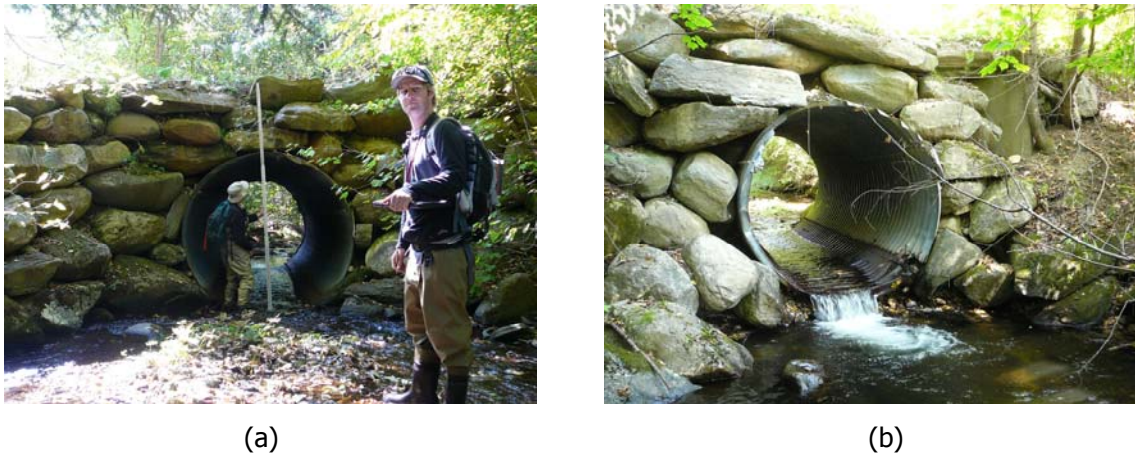
Figure 27. Instream culvert supporting driveway crossing of Twentymile Stream (M26T2.10-A) in Cavendish. (a) View downstream to culvert inlet; steep aggradational riffle partially obscuring flows. (b) View upstream to culvert outlet; 0.8-foot cascade of flow to downstream scour pool.
