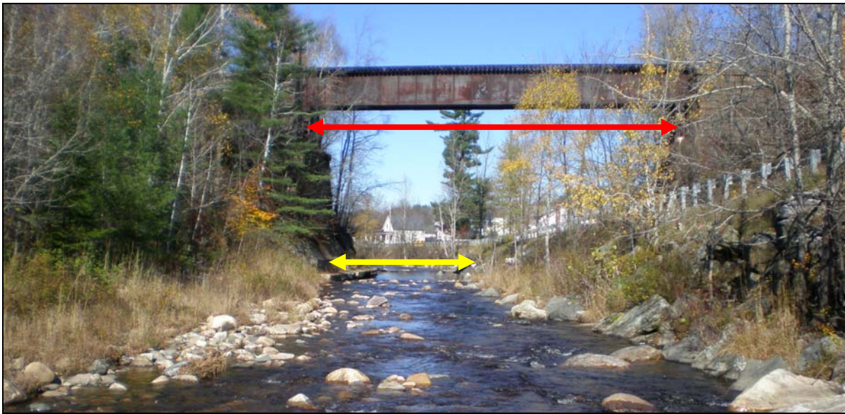
Figure 11: The railroad bridge span on M11-A is adequate for the Mill River (red line), however, location of Route 155 in relation to the bridge and the river creates a channel constriction between the bridge abutment and the road (yellow line).
