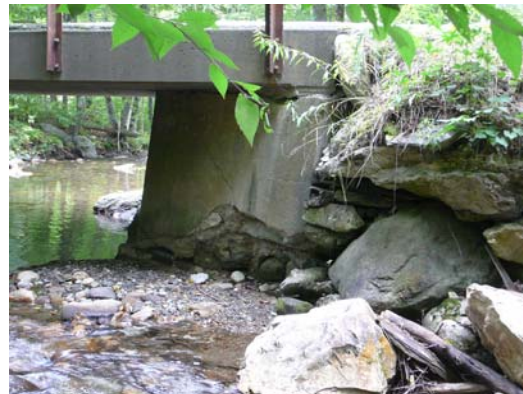
Figure 26. Scout Camp Road bridge, Segment B, M41T6.01, Buffalo Brook, 18 September 2009. (a) View downstream, to sharp approach angle, sediment accumulation at the inlet, armored banks, stepped footers on LB abutment. (b) spalling, cracking and apparent dislodging of right bank abutment.
