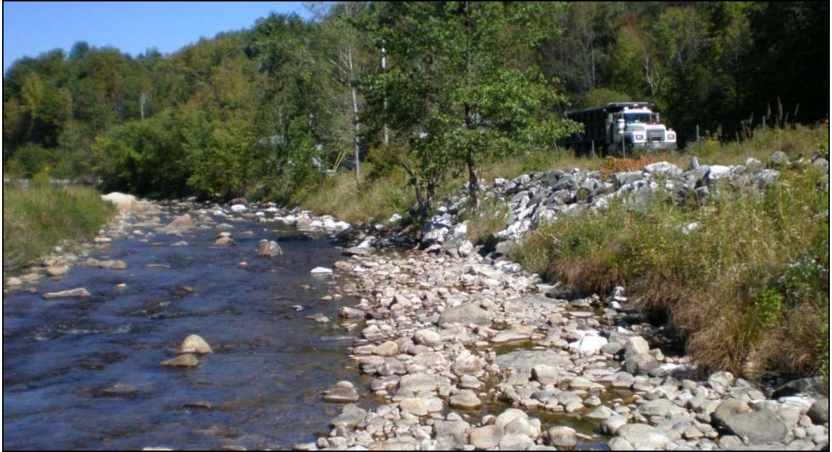
Figure 16. M06 flows through Cuttingsville and has been significantly impacted by channel straightening, armoring, berming, and floodplain development.
