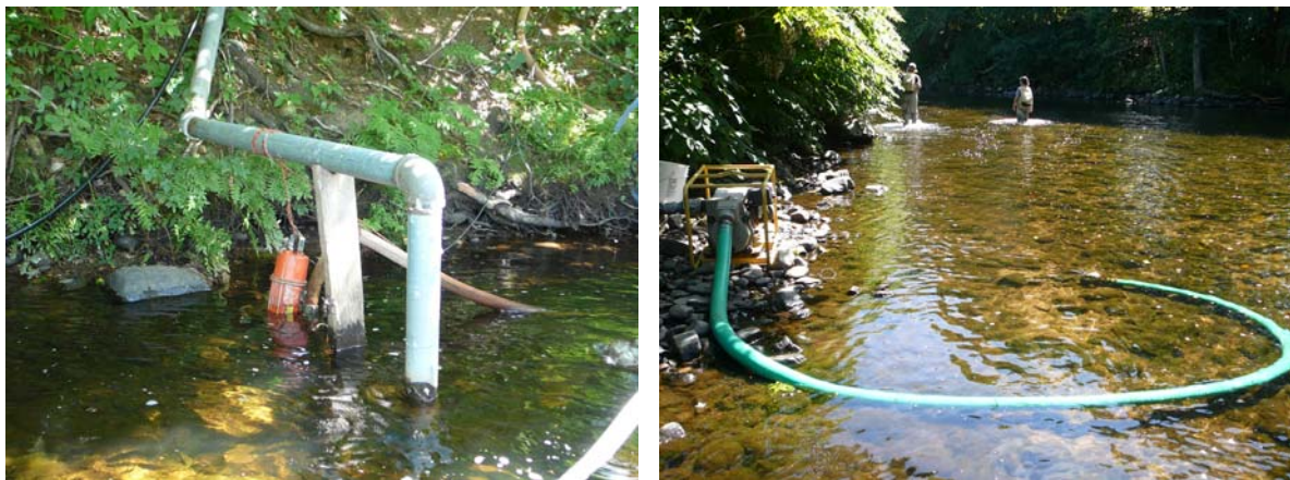
(a) (b) Figure 8. Irrigation withdrawals from Black River reach M36 (Segment B) direct water to an irrigation pond at the Okemo Valley Golf Club. (a) upstream withdrawal point; (b) supplemental (?) withdrawal approximately 200 feet downstream. 27 August 2008. Given the proximity of these two withdrawal points and the fact that they appear to both be directed to the same irrigation pond, they were indexed as one single withdrawal.
