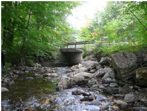
Figure 26. Scout Camp Road bridge, Segment B, M41T6.01, Buffalo Brook, 18 September 2009. (a) View downstream, to sharp approach angle, sediment accumulation at the inlet, armored banks, stepped footers on LB abutment. (b) spalling, cracking and apparent dislodging of right bank abutment.
