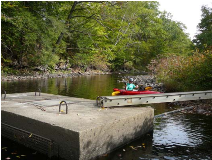
Figure 13. Water withdrawal intake structure for Okemo Mountain snow making located on the Black River (reach M34). An inflatable dam/ weir and flume apparatus for monitoring flow rates on the Black River during snowmaking withdrawals is located approximately 150 feet downstream of this intake structure (see Figure 14). Dam not inflated on date of observation, 1 October 2007.
