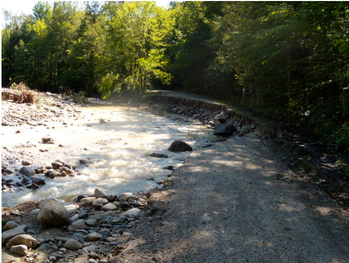
Effects of Fluvial Erosion on Freeman Brook Road
