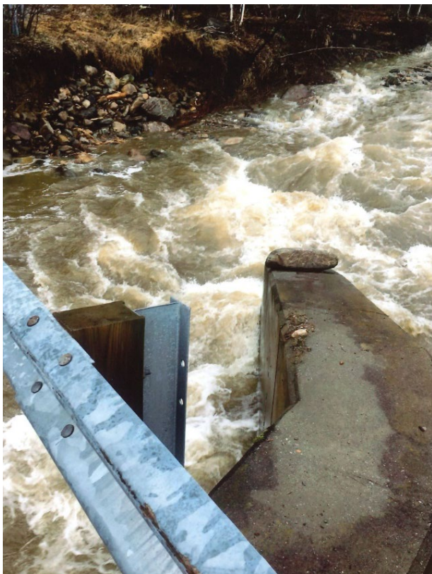
Effects of Fluvial Erosion on Lushas Acres Lane and Bridge B65 along Freeman Brook
