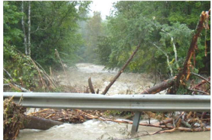
Debris Jam at Bridge (B1-2) on VT Route 155 – Tropical Storm Irene
