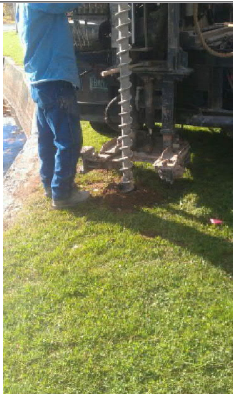
Photograph A.01 ~ View of Auger Probe 102 being drilled near the left abutment wall by Mike's Boring
