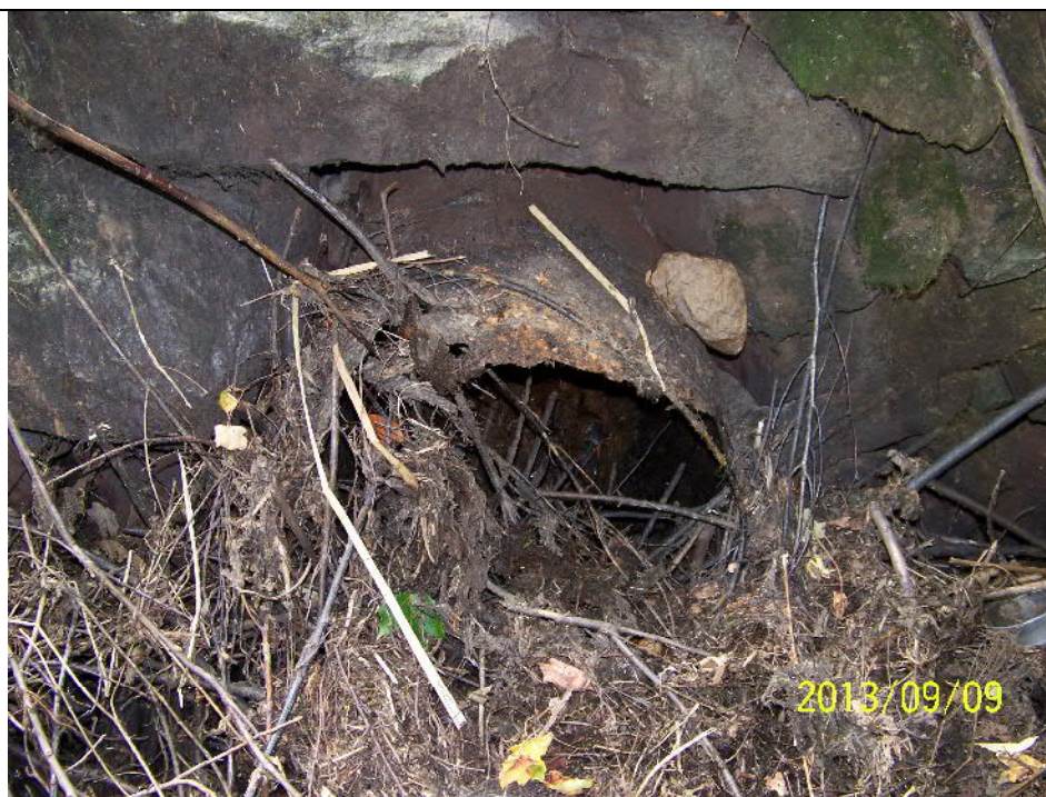
Photograph 06 ~ A view of the low level outlet located underneath the spillway.
